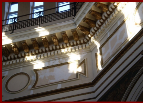
The cleaning, repair of plaster and repainting of the Courthouse Cornice has begun!
