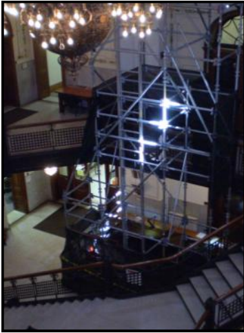
Below: Scaffolding from the bottom up.
