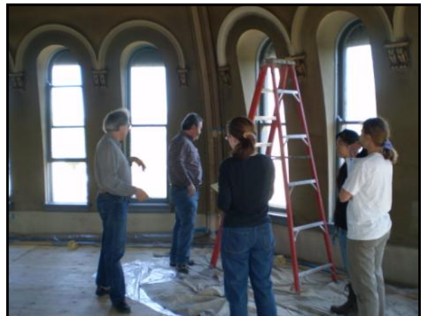
Right: Paint conservators, the architect and the Bradford County Maintenance Director discussing the progress.
