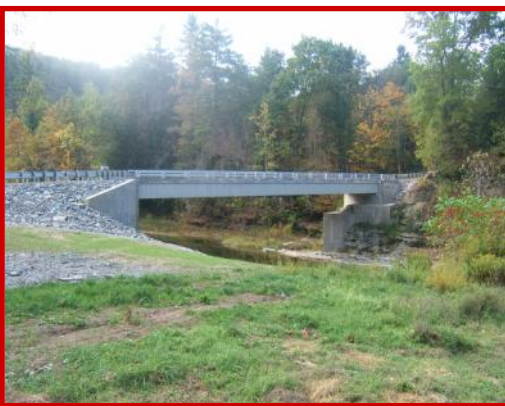
Bradford County Bridge #32 North Towanda Township
